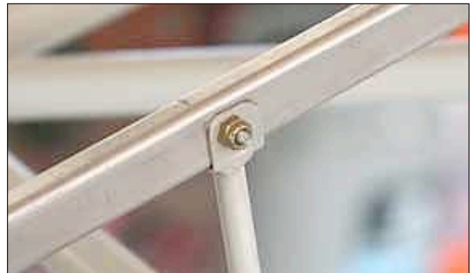
Regardless of what is used for stringer material it is important that the stringer surface be above the edges of the clips so nothing is touching the fabric.
