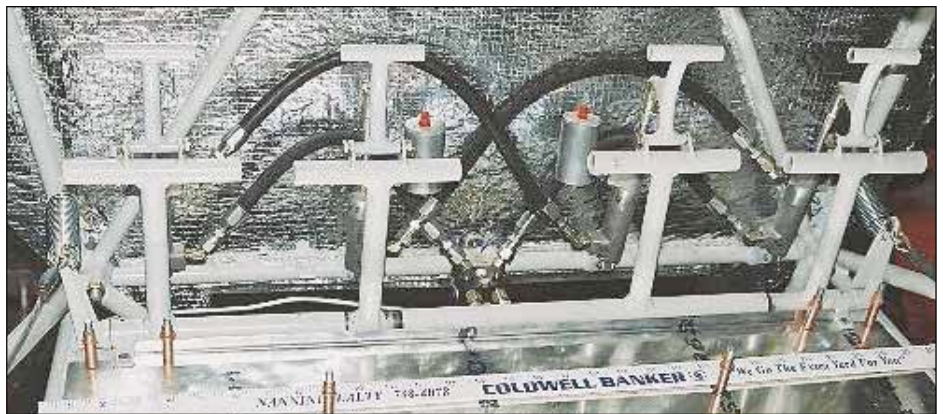
In this application the left and right master cylinders are plumbed together with the "out" lines plumbed to hard lines to the landing gear in the middle. Integral reservoirs are used on this installation.
