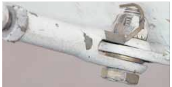
Tail strut clevis fork needs washers to keep from crushing it. This is also an excellent example of why you paint all the parts separately, rather than when assembled. Painting hardware always results in flaking paint.
