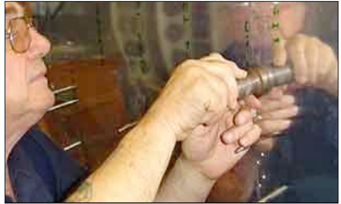
Here the back riveting bar is held against the head of the rivet.
