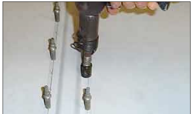
The spring loaded set on the rivet gun is used on the inside of the wing against the shop end of the rivet. The spring loaded housing holds the stiffener in contact with the wing skin.
